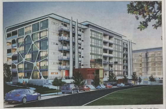
• The housing department's Adara apartments in Success were built with modular construction, keeping the cost down.
